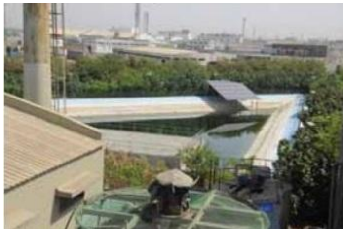
RCC offline pond
